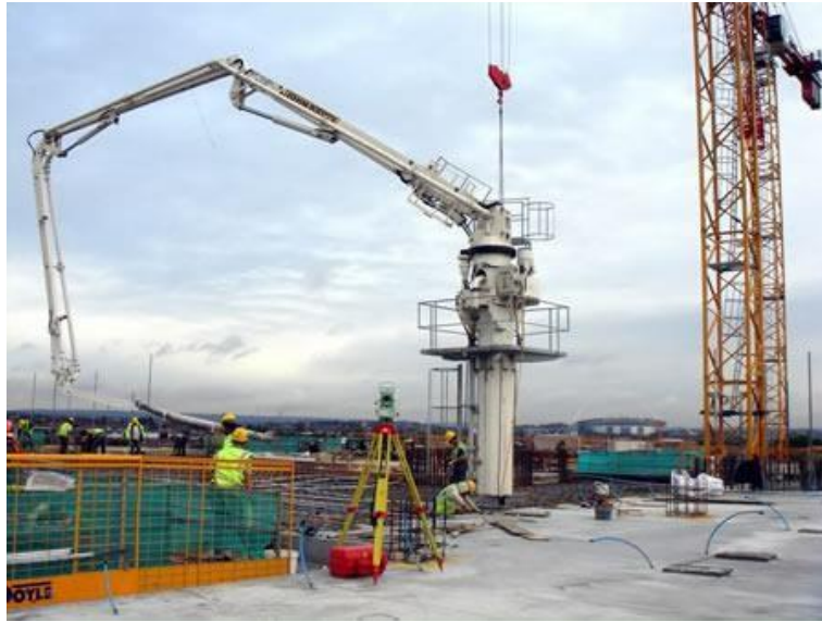
Figure 14 | Typical Concrete Placement
