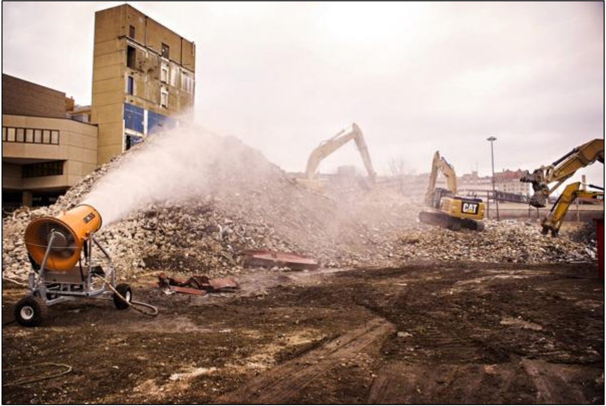
Figure 16 | Typical Dust Mitigation Measures
